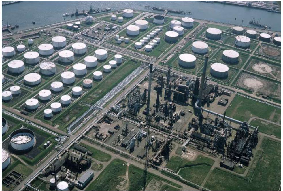
Fig 1. – Large chemical processing refineries can have over 100+ designated static earth grounding points that electricians must check on a regular basis
