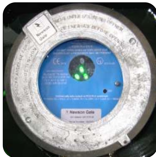
Fig. 3 Earth-Rite® PLUS ground status indicators pulse continuously when grounding is in place.
